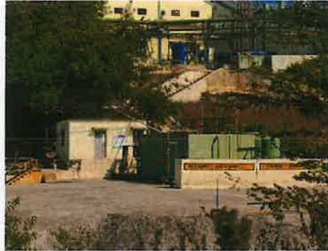
Figure 17: STP Area backfilled and paved (facing Northwest)
