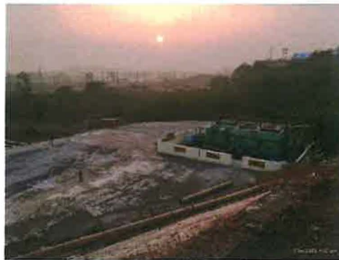
Figure 16: STP Area backfilled and paved (facing Southwest)
