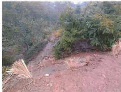
Figure 14: Northeastern edge of Miyawaki Plantation Area showing depth of backfilling
